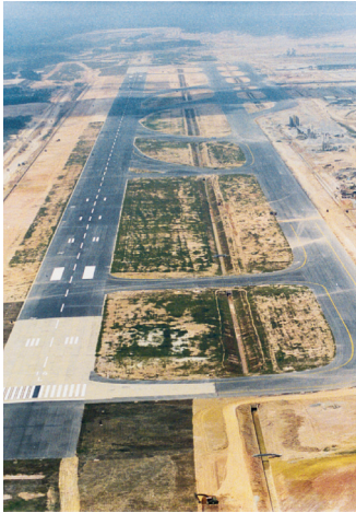
Kuala Lumpur International Airport Runway Kuala Lumpur
