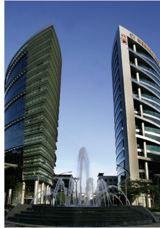
Government Administrative Office Kuala Lumpur
